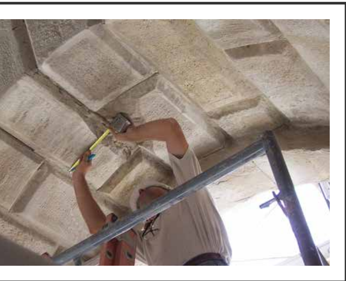
Re-anchoring terra cotta with Stitch-Ties
